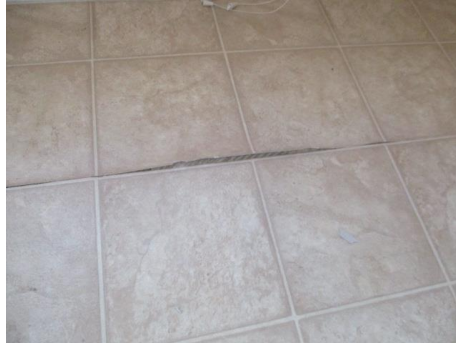
Damaged vinyl flooring in the kitchen.
