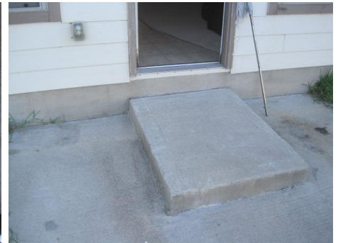
Damaged rear exterior door. Inadequate landing at the rear entry door. The master bathroom entry door is binding against the door casing. The springs on the overhead garage door are out of adjustment. Missing and damaged doorstops.
