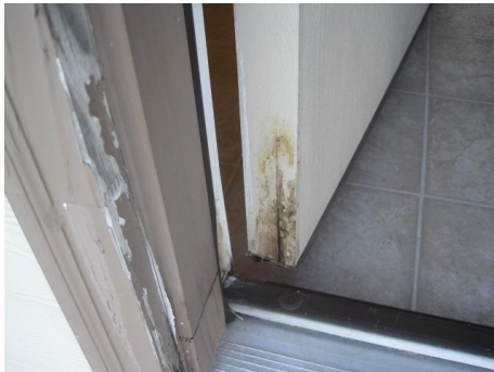
Damaged rear exterior door. Inadequate landing at the rear entry door. The master bathroom entry door is binding against the door casing. The springs on the overhead garage door are out of adjustment. Missing and damaged doorstops.
